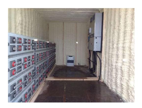
192KWH 4000AH Off-Grid Installation Using 2ndLife AGM Lead-Acid batteries Located in remote Northern Quebec
